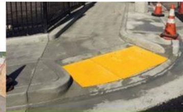
Ramp at Venice & Arapahoe
