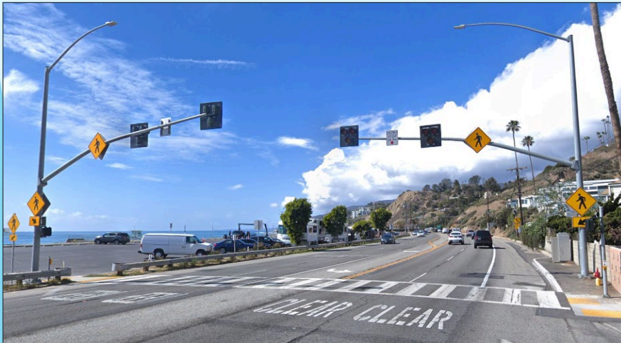
D7: High intensity Activated Crosswalk (HAWK) beacon at SR-1/ Pacific Coast Highway and Driftwood Dr., Pacific Palisades Photo Credit: Google
