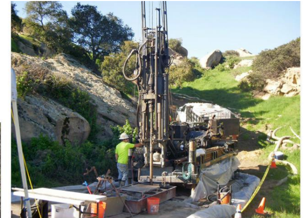
Drilling groundwater monitoring well
