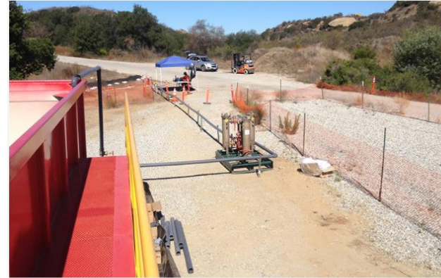
Groundwater cleanup operations
